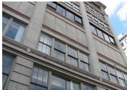
Existing concrete façade
