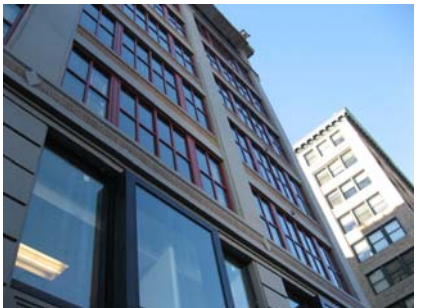
Newly coated concrete façade
